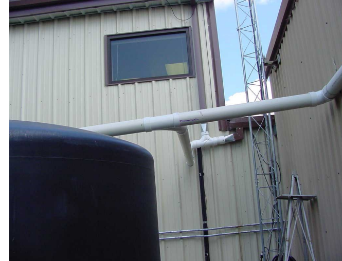
The system comes together behind the office to flow into our storage tank to be used to water our lawn and xeriscape garden.
